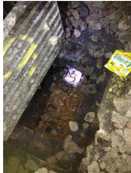
Figure 7: Informal chambers within Pill tunnel; observed as twin wall pipes with top half cut out with concrete frame and steel grate.
